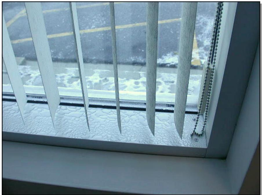
Figure 2—Condensation has formed on these exposed metal window surfaces due to wall construction that has compromised the window's design features.
